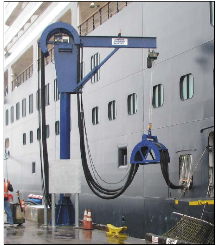
Cruise ship connected to the Port shore power system.
