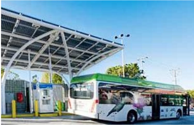
Emeryville: H 2 from solar electrolysis and liquid delivery
